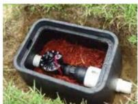
Always install downstream from all shut off valves.
